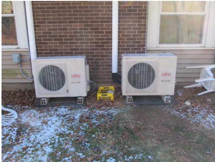
Typical exterior condensers for heat pumps recently installed in all units
