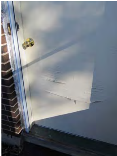
Wear/damage noted on exterior surfaces at several unit entry doors
