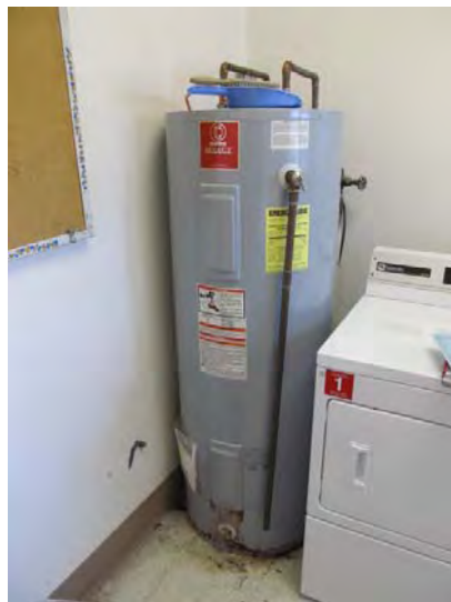
Electric, storage-type, domestic hot water tank for common areas at community building
