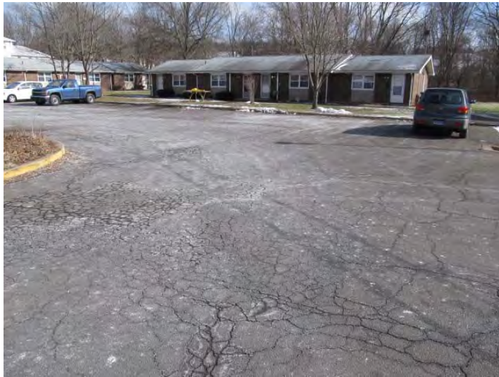
Cracks and alligatoring evident at parking area asphalt paving
