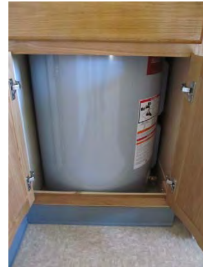
Each unit has its own electric, storage-type, domestic hot water tank
