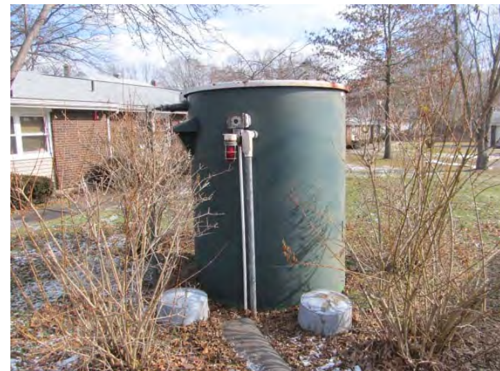
On-site, duplex-type, sewage ejector pump system serving the development
