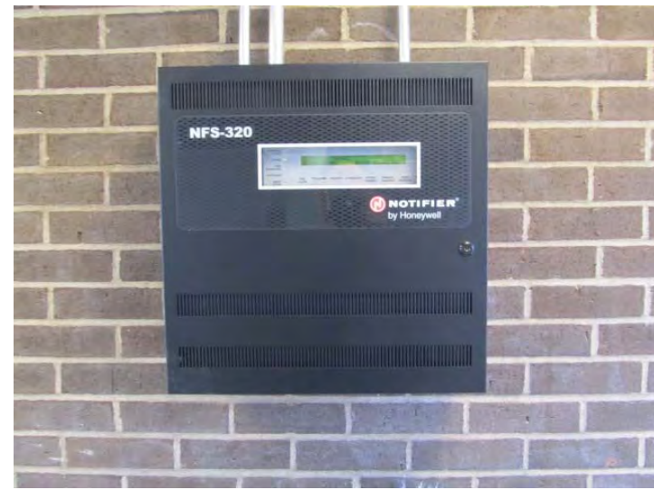
Recently completed development wide fire alarm system upgrade includes this fully addressable control panel located at the community building
