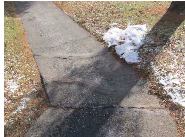
Cracks/tree root damage at pedestrian walkways pose potential trip hazards
